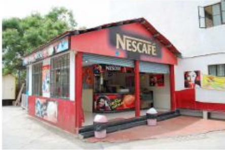
No. of Cafeteria Hall and Size: 04 and 150 Sqm
